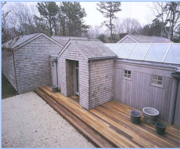
Above, the entrance to the house, seen from the first floor, resembles a gatehouse, completely covered with cedar shingles. On the right the exterior of the long corridor with its glazed roof which links up the various parts of the house. The front perron is made in mahogany. Below, the view of the entrance and the right wing of the house where the guest accommodation is located.
