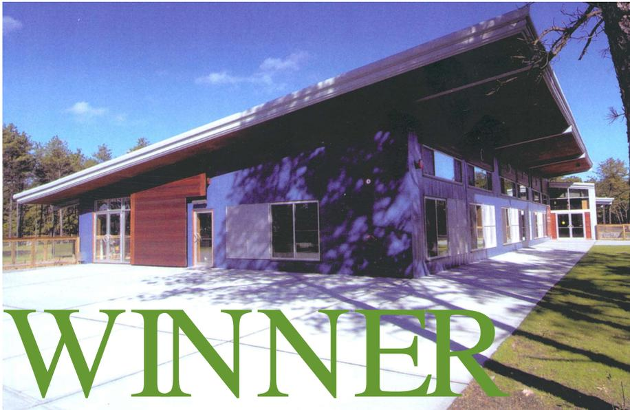
**About the products:** At the heart of the buildings construction is a 180' x 69' single - sloping clear span framing system with a 2:12 roof slope. It features concealed gutters, hidden fasteners, alternating pitches and a roof system that wraps down to become the walls in some areas. Kirby Building Systems manufactured the framing and roofing while Jenisys produced the metal wall panels.
